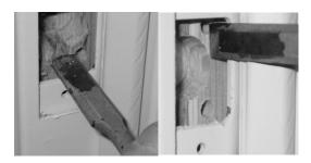
**10.** Clear out the remaining wood with a wood chisel. Note: Step 9 & 10 may be easier done before complete installation of pre-hung frame assembly.
