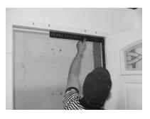
**4.** Remove pre-hang clip and open door. Use a carpenter's square to square header to hinge jamb. Install one drywall screw in center of header.
