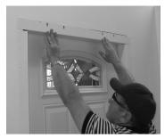
**7.** Slide header closure trim into header. Adjust vertical and header closure trims to obtain a good fit in the top corners.
