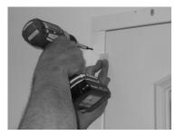
**5.** Close door and secure strike jamb using a 1/8" spacer to obtain a consistent gap as you work toward the bottom. Install remaining screws in header.
