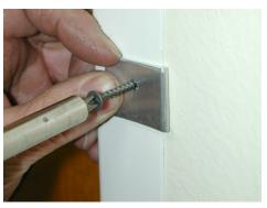
1. Examine retainer clip. One side has an undercut 1/8" from edge. Position clip on frame with undercut tight to edge of frame and with the hole lined up with the hole in frame. Secure with #6 x 1-5/8" bugle head screw. Repeat for all remaining holes in frame. 6 clips on each jamb and 3-4 clips on header depending on width.
