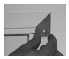
3. Insert casing corner brackets into header.
