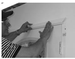
**2.** Position header casing over top edge of clips and center. Tap casing toward door near each clip to snap it over the clips.
