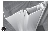
On the other side of door, slide the jamb closure trims into the jambs, starting from bottom.
