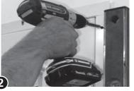
Use a level to plumb hinge jamb. Secure near top corner with a drywall screw.
