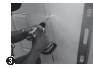
Install screws in the hinge iamb, start at top, checking for plumb as you work to bottom.
