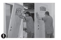
Place bottom of door unit in bottom of opening. Lean top of door away from wall. Have helper caulk bottom of sill. Stand door upright, centered in opening and against wall.
