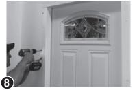
closure trim near the top corners. Then install the remaining screws.
