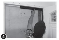
Remove prehang clip and open door. Square header to hinge jamb. Install drywall screw in center of header.
