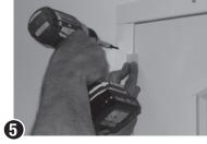
Close door and secure strike jamb using a 1/8" spacer for a consistant gap thru bottom - Install remaining screws in header.
