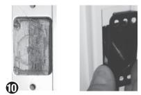
Clear out remaining wood with chisel. Test depth and clearance with the plastic deadbolt strike box.
