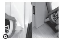
Allow caulk to set before reinserting weatherstrip. Caulk outside sill and closure trim to floor. For exterior. caulk frame to closure trim at jambs & header (as arrow indicates).
