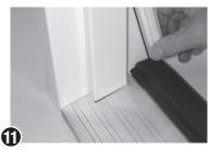
Pull weatherstrip out of the kerf near sill to allow room for caulking. Install sill extender if required.
