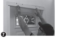
Slide header closure trim into header. Adjust vertical and header closure trims for a good fit in top corners.
