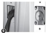
Prepare stud for deadbolt clearance. Bore a 7/8"-1" hole to a depth of 1" from face of frame. Drill a 3/8" diameter hole at corners - 1" from face of frame.
